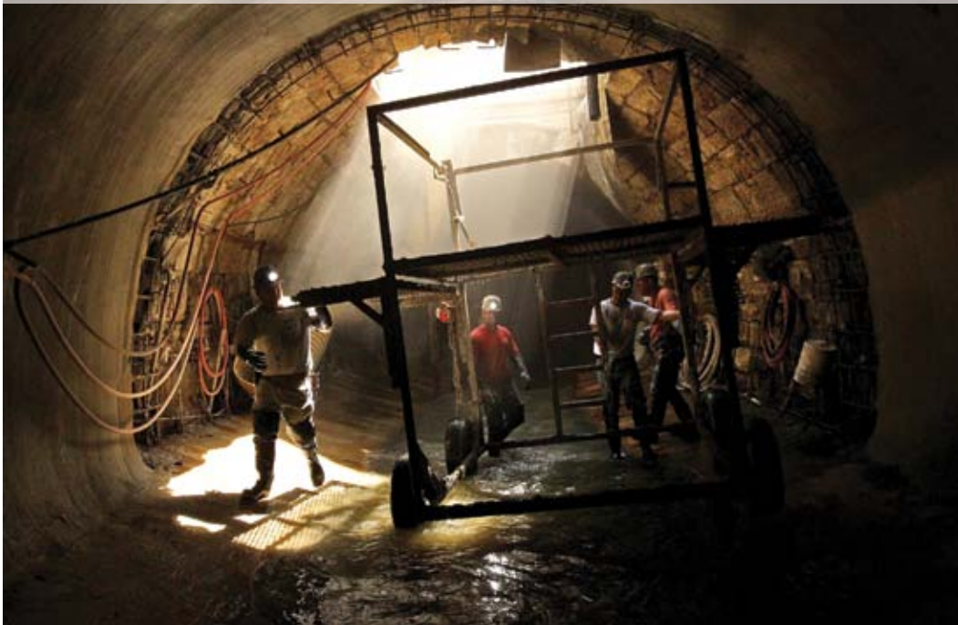
Workers restore a section of storm sewer about 25 feet below ground in St. Louis, Missouri.
