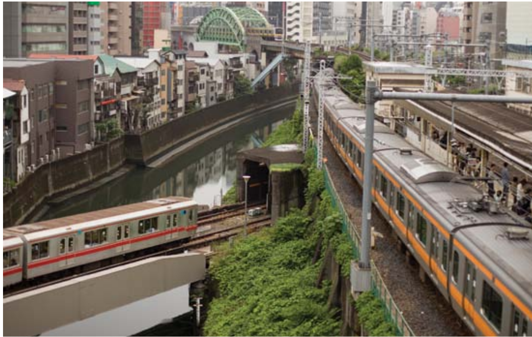
Japan has made significant investments in trains and other urban infrastructure.
