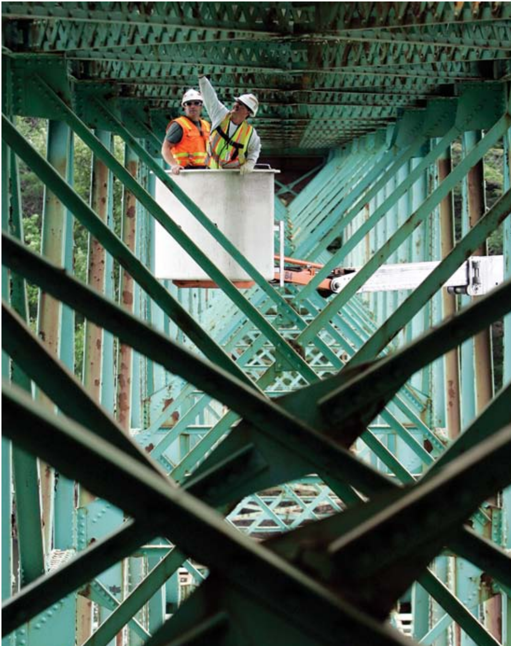
Bridge inspectors check the condition of the Back River Bridge in Georgetown, Maine. (©Associated Press / Robert F. Bukaty)
