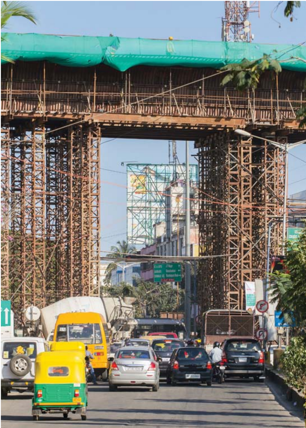
Steel scaffolding for construction of the Bangalore metro rail rises above a street in south Bangalore, India.
