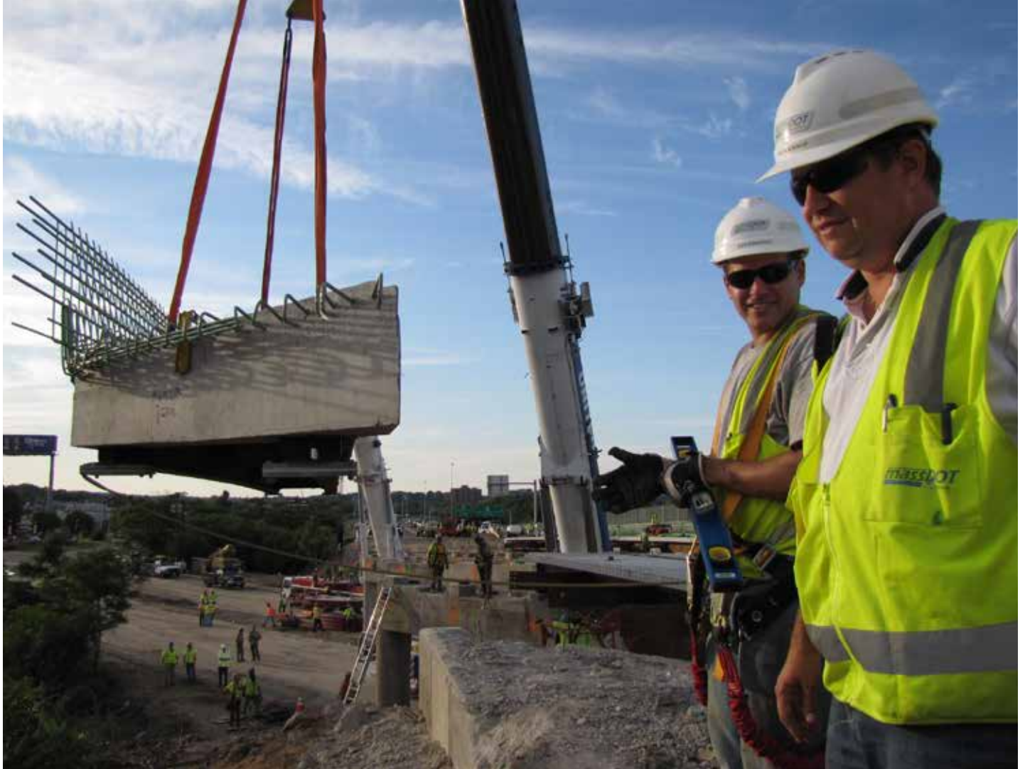
MassDOT construction inspector Alex Normandin and Assistant Resident Engineer Bob Blackmar on August 13, 2011, as one of the 94 Fast 14s 252 Prefabricated Bridge Units is lowered into place. MassDOT used this innovative method of construction to maximize mobility while safely replacing fourteen Boston-area bridges in just 10 weekends. Photo courtesy of Massachusetts DOT. Photographer: Eliza Partington.
