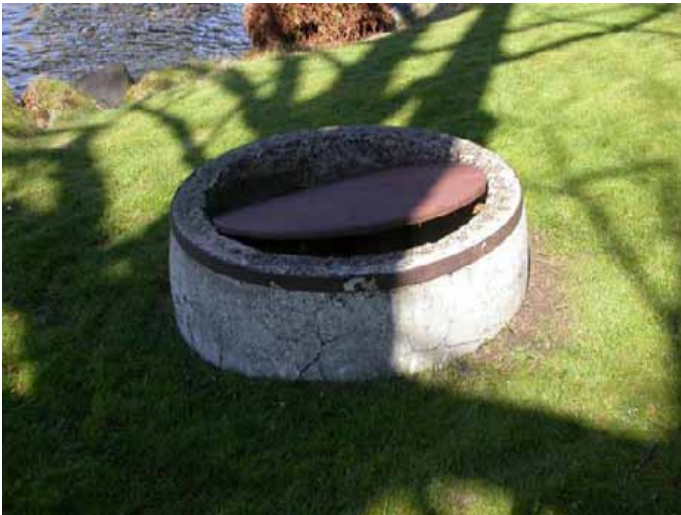
View of Remains of well/cistern, west of main house, near water's edge taken 3/8/2004
