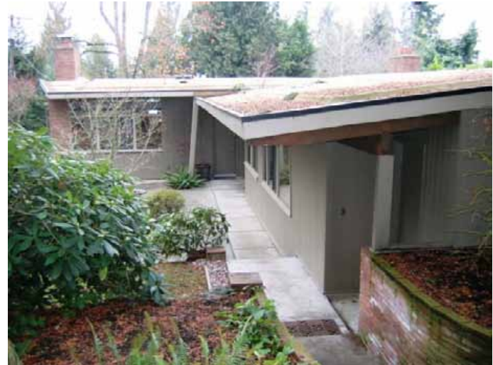
View of east and south elevations taken 1/22/2009
