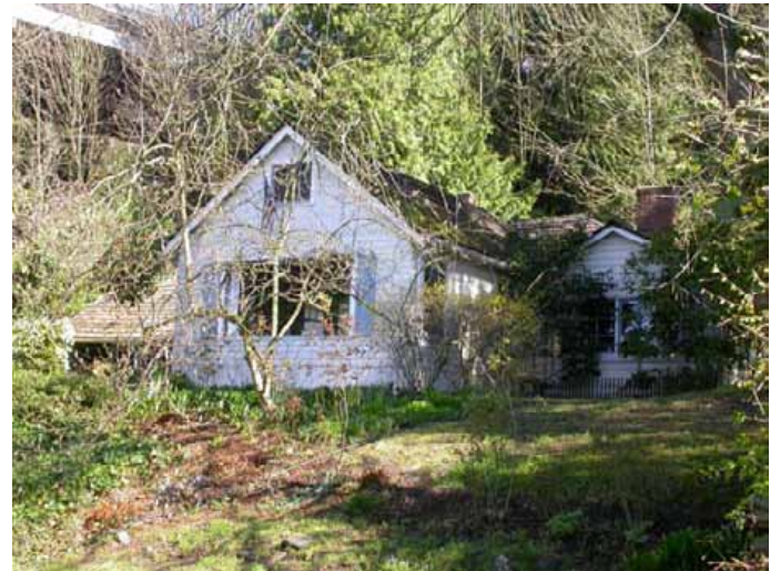
View of West and south elevations taken 3/8/2004
