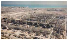
Liquefied natural gas processing facilities condense natural gas for transport to global markets. The facilities constructed today are more than 20 times larger than the first ones built in the 1960s.
