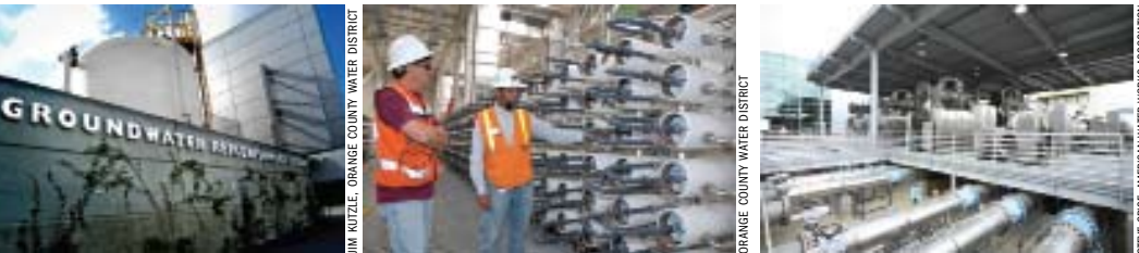
In California, demand for the state's limited water supply has resulted in a groundwater replenishment system (GWRS) for Orange County's Water District (above). The GWRS purification process includes reverse osmosis (above right) and ultraviolet light with hydrogen peroxide for advanced oxidation (above far right).
