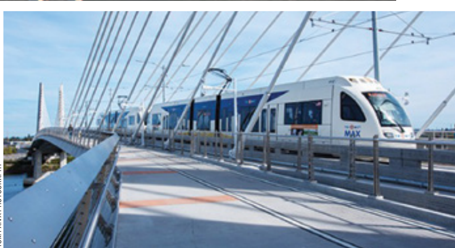
The Tilikum Crossing Bridge over the Willamette River in Portland, Oregon, carries transit (below) and pedestrian traffic. The bridge is designed to withstand a seismic event such as a 9.0 earthquake along the Cascadia Subduction Zone.
