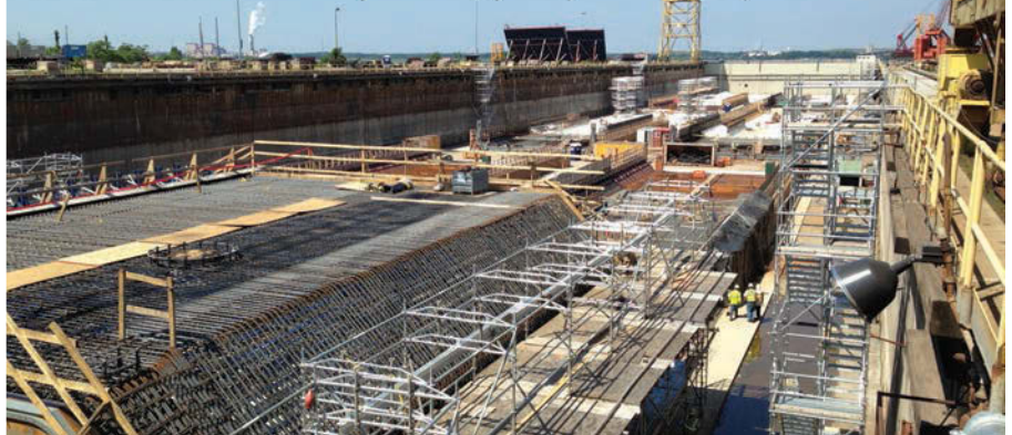
WSP | Parsons Brinckerhoff designed the Second Midtown Tunnel, which will double traffic capacity across the Elizabeth River between Norfolk and Portsmouth, Va. The project is part of a $2.1 billion P3 between Elizabeth River Crossings and the Virginia Department of Transportation.
