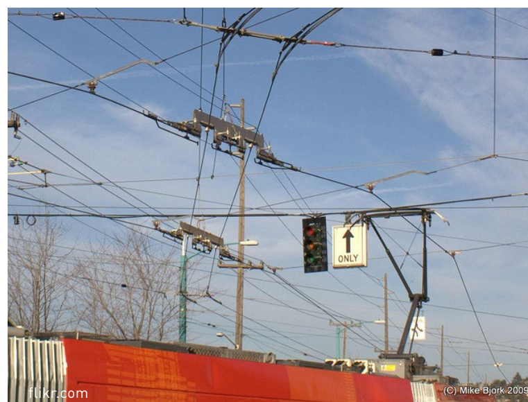
South Lake Union Streetcar Catenary (overhead wire) System
