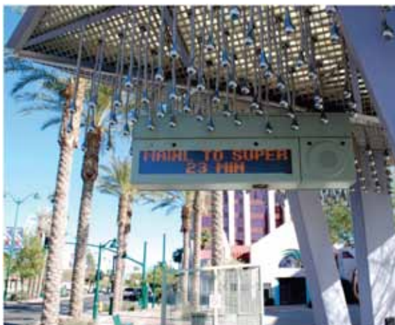
FIGURE 24 Mesa (Arizona) BRT station DMS (Courtesy: TranSystems 2011).
