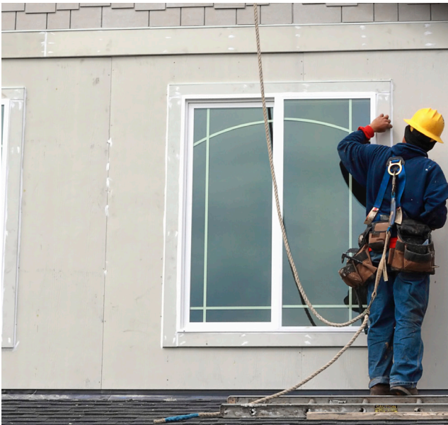
Figure 1.6: The installation of 99 million windows, 45 millions square feet of window wall, and 31 million square feet of curtain wall will create 2,700 construction jobs each year from 2015 to 2050.
