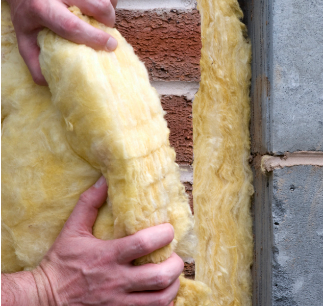
Figure 1.4: 6,500 construction workers 5 will be needed each year from 2015 to 2050 to install a total of 5.7 billion square feet of insulation to building roofs and walls.
