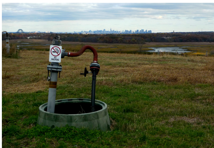
Figure 7.2: Methane capture vent at Freshkills Park, a landfill reclamation project in Staten Island.
