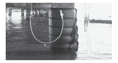
**Figure 1** *Pressure bagging for enhancing FRP-concrete bond*
