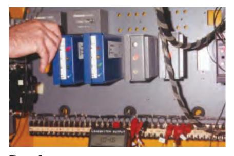
**Figure 1** Installation of conservation load switch in standard cabinet.
