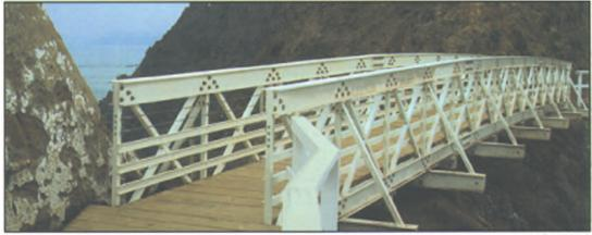
**Figure 1** *E. T. Techtonics composite pedestrian bridge.*
