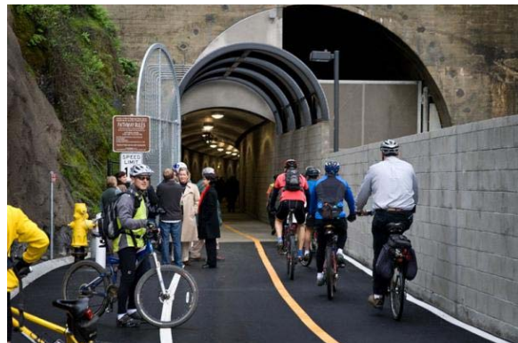
Figure 21: Cyclists in Tunnel at North Portal (source: WalkBikeMarin)
