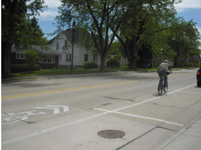
Figure 37: The New Sidewalks and Bicycle Lanes along South Main Street Provide Safe Spaces for Bicycling and Walking (source: Sheboygan County NOMO)
