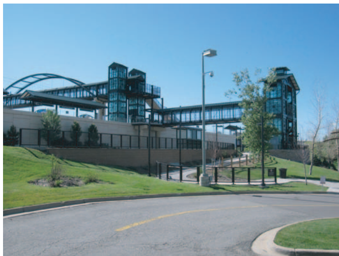
Exhibit 7-2. Pedestrian ramp providing station access (County Line RTD Station, Englewood, CO).
