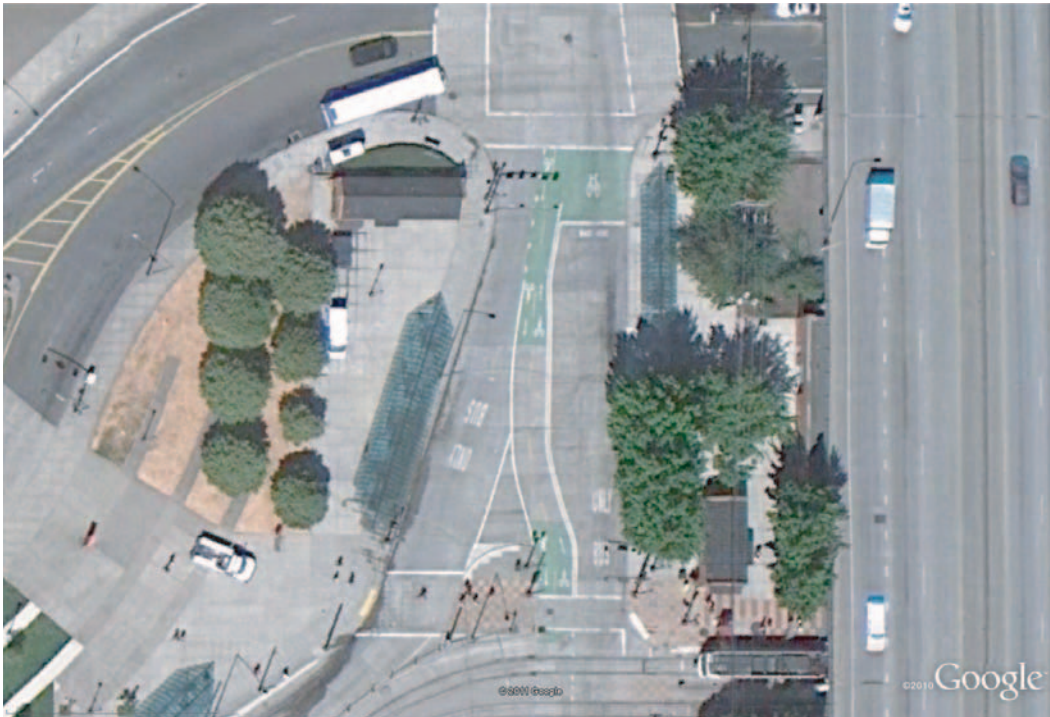
Exhibit 8-5. Bicycle facility through the Rose Quarter Transit Center (Portland).
