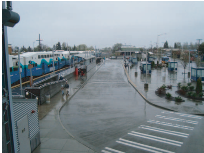
Exhibit 9-3. Feeder bus connections located close to station platform (Sound Transit Commuter Rail Station, Kent, WA).
