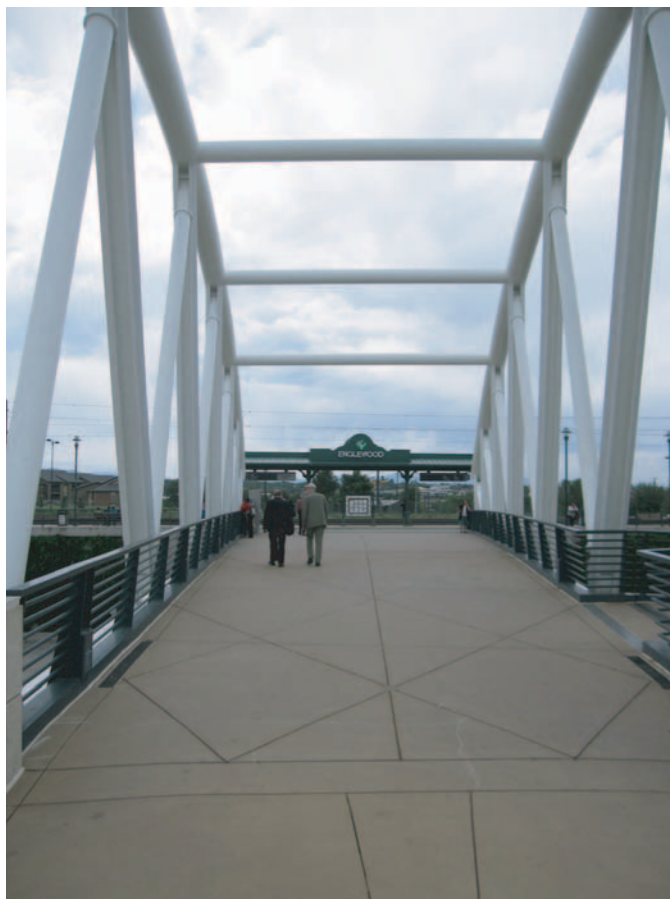
Exhibit 10-18. Direct and open connection to transit station (Englewood, Colorado).
