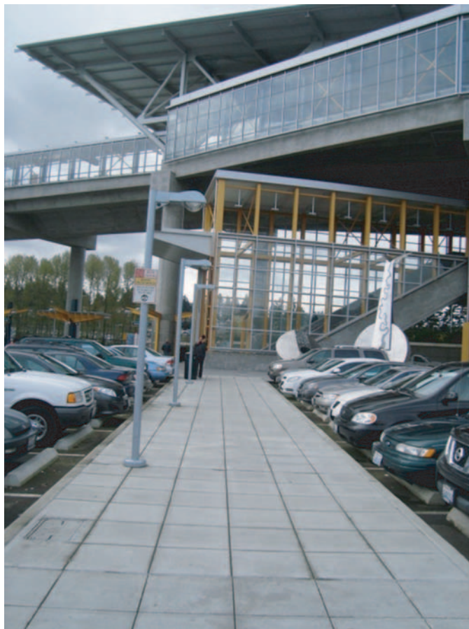
Exhibit 7-4. Example of a pedestrian route through a station parking area (Sound Transit Tukwila Light Rail Station, WA).
