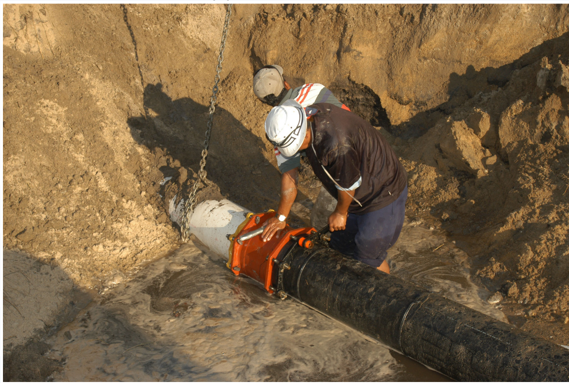
Workers install a new water pipe.
