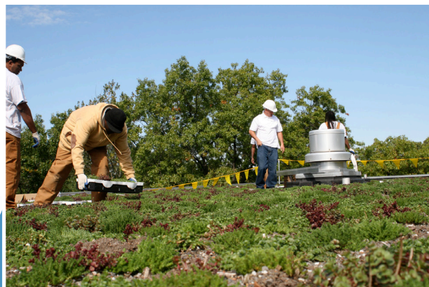
A green roof.
