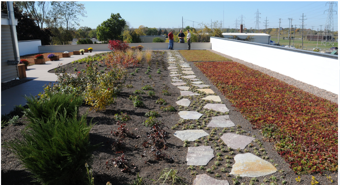
A green roof.
