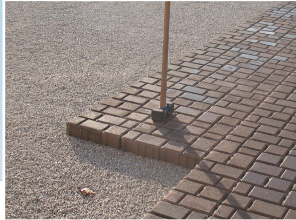
A permeable street surface.
