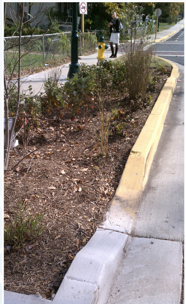
Bioswale on Maryland street capable of receiving stormwater runoff.
