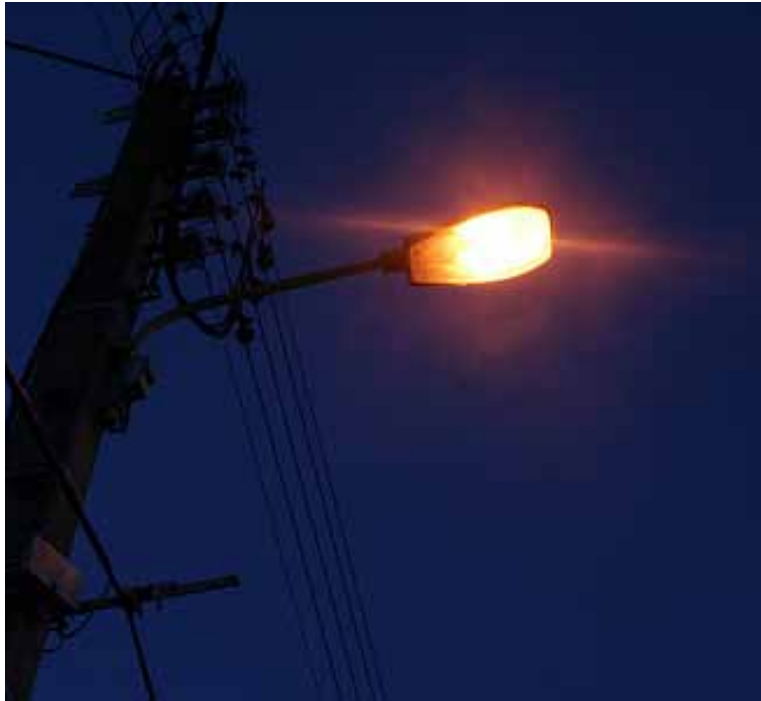
High pressure sodium light
