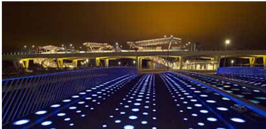
LED lighting embedded in pedestrian bridge
