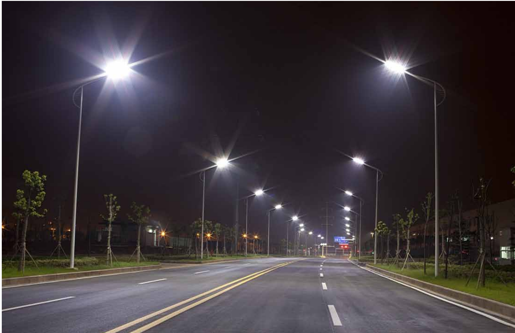
Glare produced by LED streetlights as a result of poor fixture design
