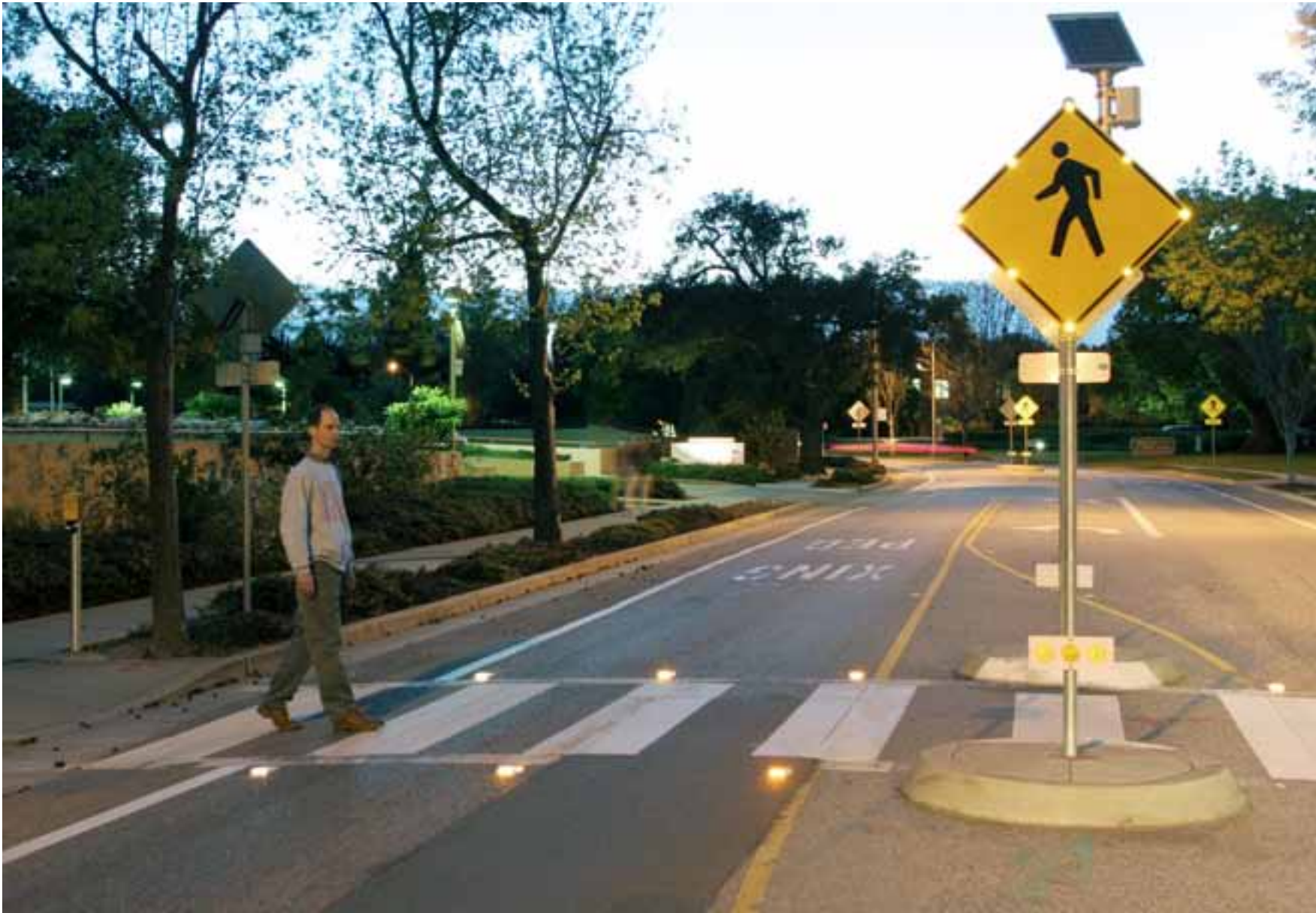
LED lights for pedestrian crosswalk
