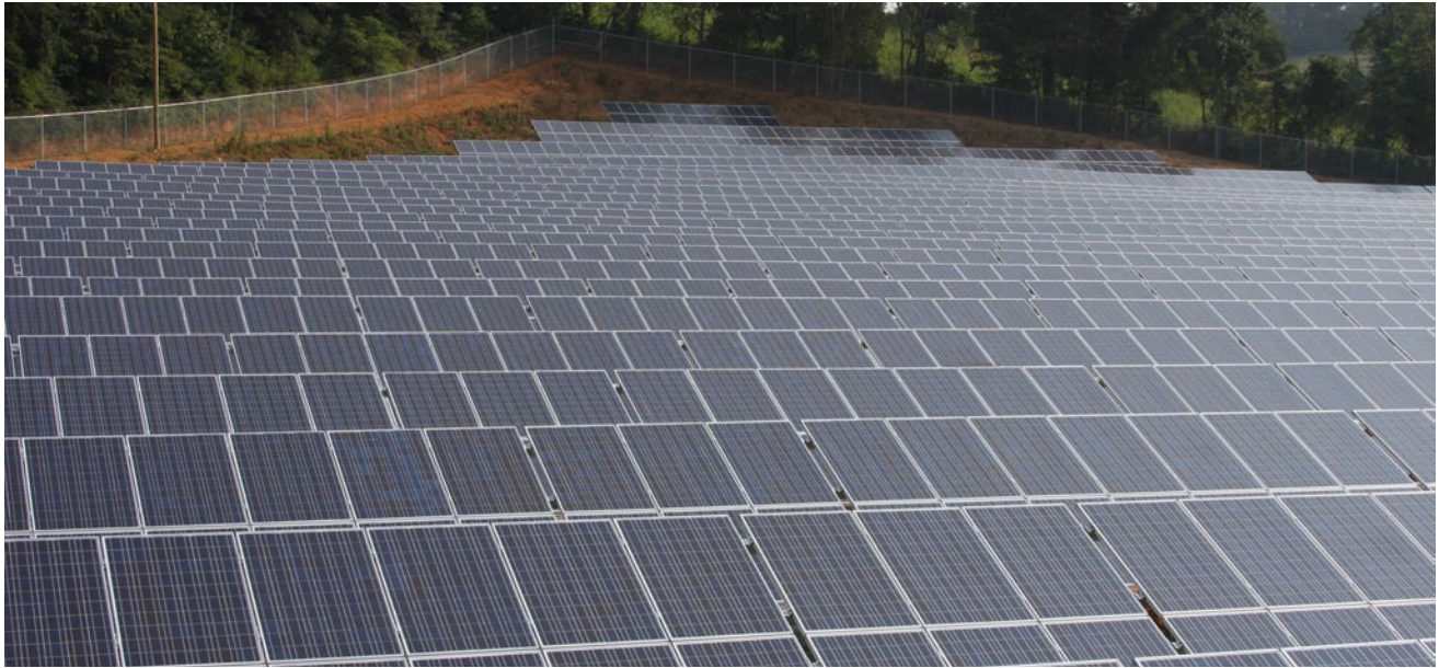
Solar panel system of the Natural Energy Group in Knoxville, Tennessee. The photovoltaic system, the largest in Tennessee, uses 4,608 Sharp modules manufactured in the state and is capable of producing 1 MW of electricity. Photo courtesy of flickr user Harvey Abouelata via Creative Commons License.
