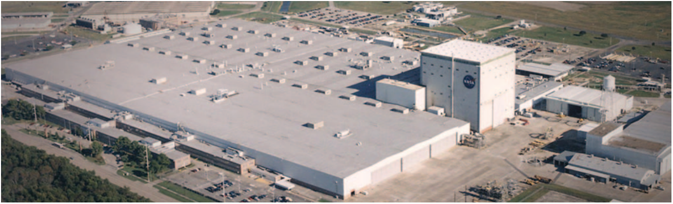
Blade Dynamics assembly facility in New Orleans, Louisiana. Photo courtesy of Blade Dynamics.
