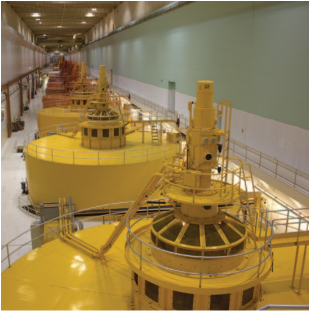
An example of hydroelectric generators, from the Dalles Dam on the Columbia River Gorge, Oregon. Photo courtesy of flickr user Sam Churchill via Creative Commons License.
