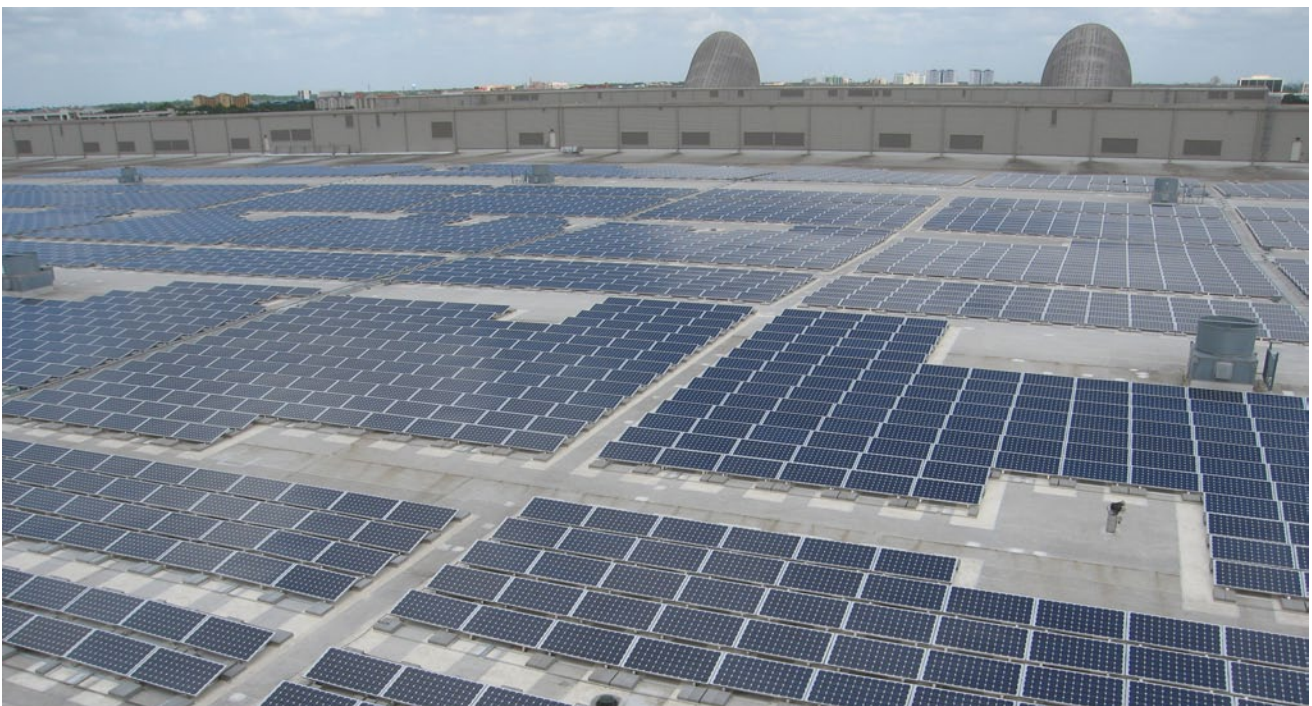
Solar photovoltaic rooftop system installed by Solar Source at the Orange County Convention Center in Orlando, Florida. Photo courtesy of U.S. Department of Energy, Office of Energy Efficiency and Renewable Energy
