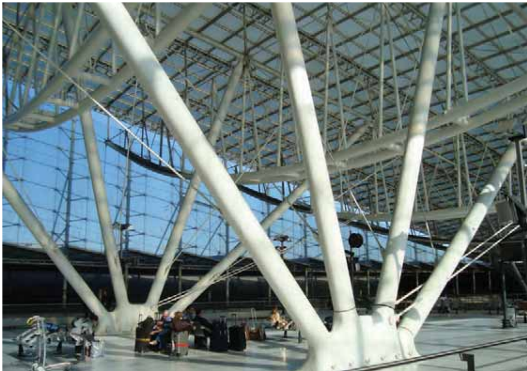
TGV Station at Charles de Gaulle Airport in Roissy, France
