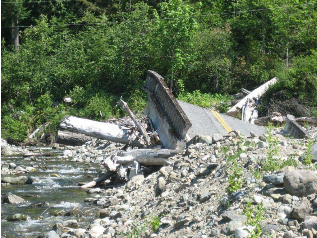
Scour and damage to structures, US-12 Davis Creek. (Photo courtesy of Washington State DOT.)
