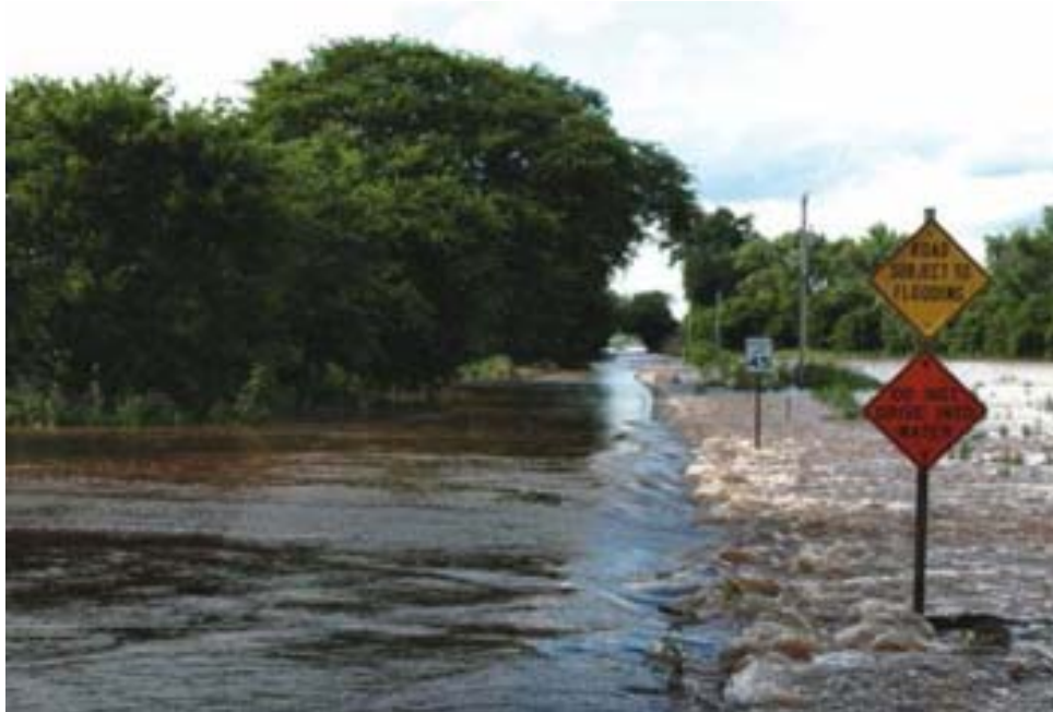
FIGURE 1 The anticipated effects of climate change on transportation include roadway flooding. (Photo courtesy of U.S. Global Change Research Program.)
