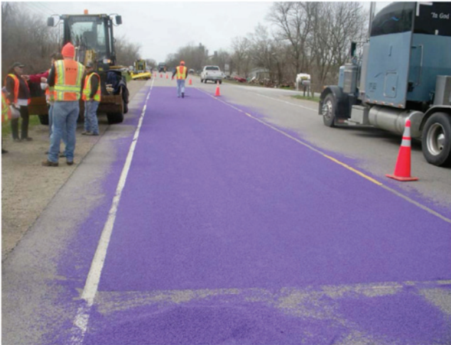
FIGURE 18 Colored pavement [Source: Russell and Godavarthy (2010)].
