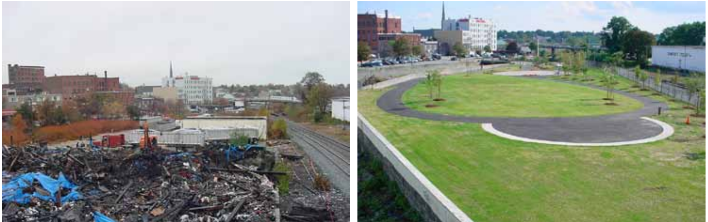
HOPE RUBBER PARKING LOT AND INDUSTRIAL WASTE SITE TRANSFORMED INTO A LUSH RIVERFRONT PARK IN FITCHBURG, MASSACHUSETTS
