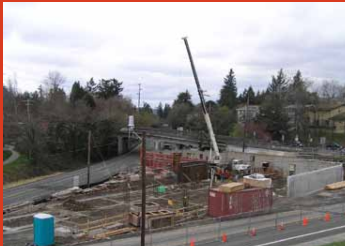
THE WATERSHED SITE UNDER CONSTRUCTION
