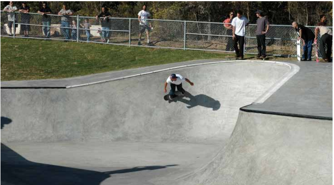
MABEL DAVIS SKATE PARK BUILT ON A CLOSED LANDFILL IN AUSTIN, TEXAS
