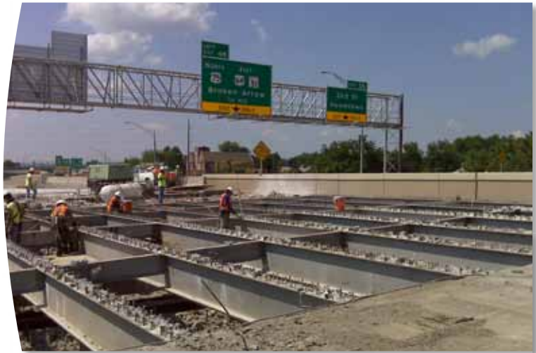
The single largest Recovery Act project in Oklahoma, the Tulsa Inner Dispersal Loop project, will replace the decks on 40 bridges.
