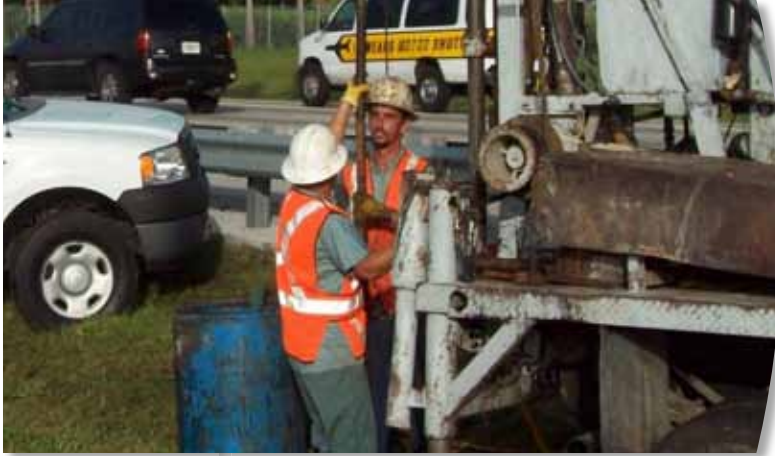
Workers take soil borings along high-speed rail route in Florida.
