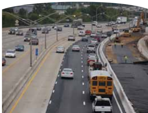
Left: Ten bridges on Interstate 96 in Detroit received new driving surfaces because of the Recovery Act.
