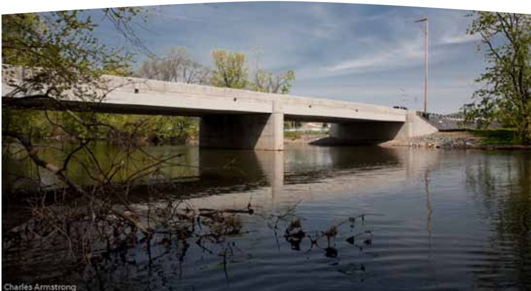
The Spring Road Bridge in Pennsylvania was originally constructed in 1930 and badly in need of replacement. © Charles Armstrong
