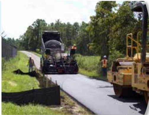
Work on the Suncoast Trail project in Florida allowed the primary contractor, Ajax Paving, to increase the hours of its workers.
