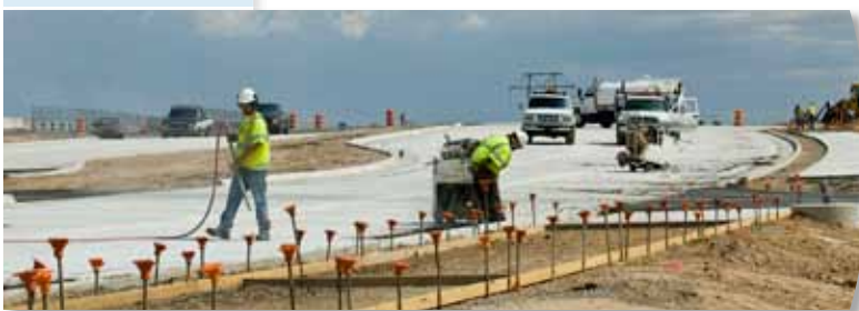
New road leading to Paseo del Volcan in New Mexico being constructed.
