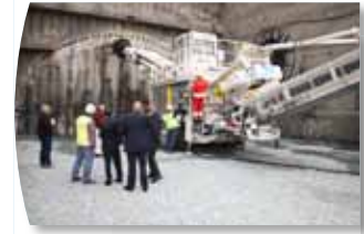
A tunnel boring machine begins work on the $420 million Caldecott Tunnel project in February.
