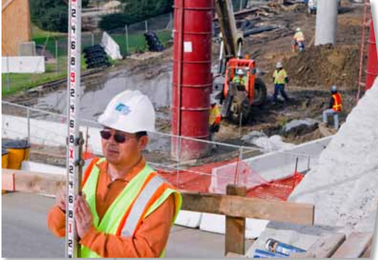
Worker at the site of the Chester Avenue Bridge reconstruction in California.
