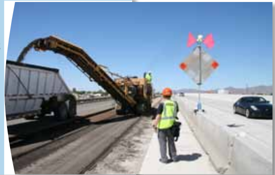
Crews remove old asphalt pavement as part of a $22 million Recovery Act project to reconstruct and widen a busy section of Interstate 10 in Arizona.
