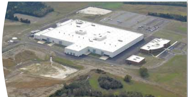
Newly constructed Paccar manufacturing plant in Columbus, Mississippi.
